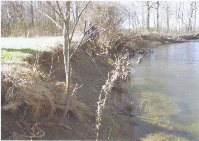
INITIAL: Severe bank erosion
